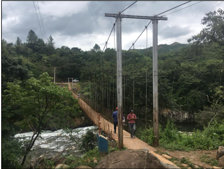
Figure 4. Suspension Bridge in Llano Ñopo
